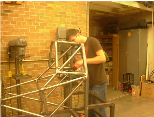
Vladimir finishing some of the welds
